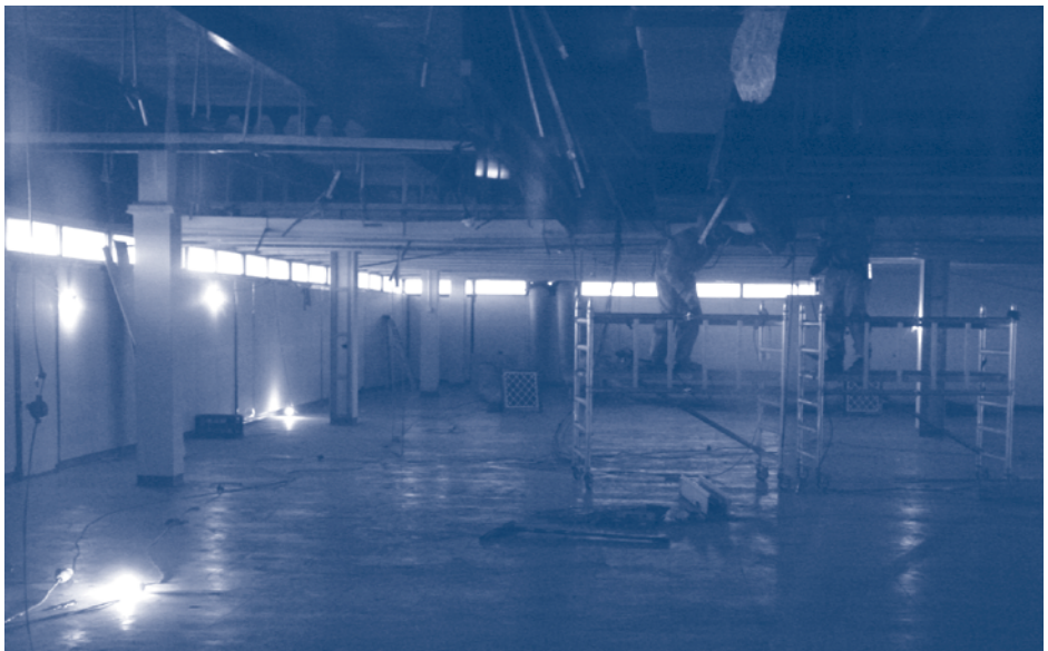
Main Library sixth floor: being gutted for a completely fresh start
