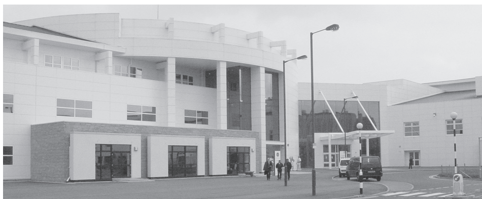
The Medical School at the New Royal Infirmary. The statistics of its network are impressive: there will be over 400 telephone points, and some 3,000 active 10/100Mbit/s data outlets, supported by 65 Ethernet switches connected in a star network to a core Cisco Catalyst 6509 via Gigabit-Ethernet connections. The copper cabling is estimated to be over 170km long, and to weigh some seven metric tonnes. The network is due to be in full operation by the end of May. See for yourself, at the superb http://www.med.ed.ac.uk/location/eri/map.htm
